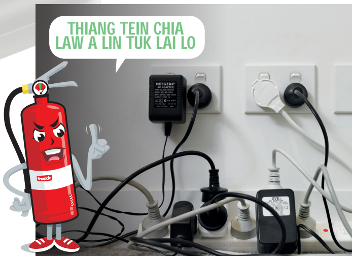
Lektrik lei meihri cu a awngkua pakhat ah hri pakhat lawng sawh. Meitunnak kuang pawl kha a tamtuk hmang hlah. Meihri sawhnak pakhat a umnak ah 'aa thuahin' 'piggyback' in sawh hlah asilole pehtlaihnak pahnih a ummi hmang.
