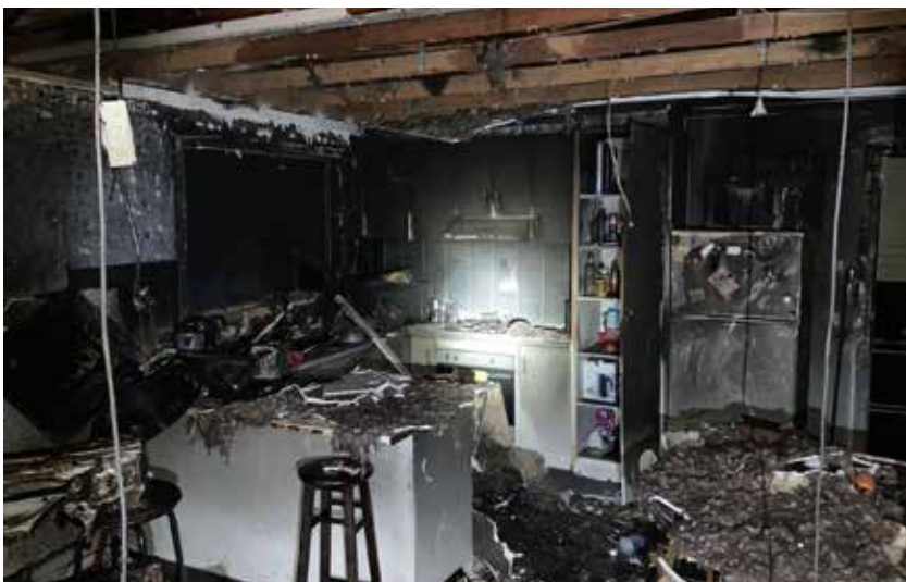
Clockwise from top left: Fire in bedroom caused by overloaded electrical equipment including lithium ion batteries. Fire in kitchen caused by defective scooter battery.
